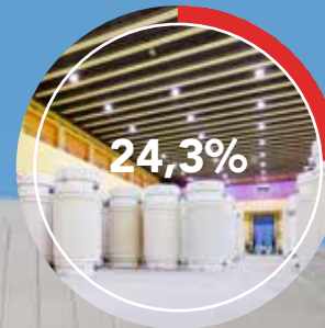
Interim Storage Facility Würenlingen AG (Zwilag) Direct shares Axpo Power (excluding indirect shares through partner plants of KKL and KKG)
