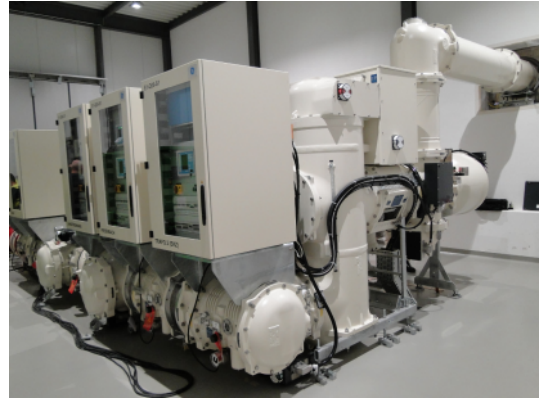
Left: The new Etzel substation in Altendorf (SZ) on an area of about 600 m 2 . Right: The compact, gas-insulated switchgear using the climate-friendly gas g3.
